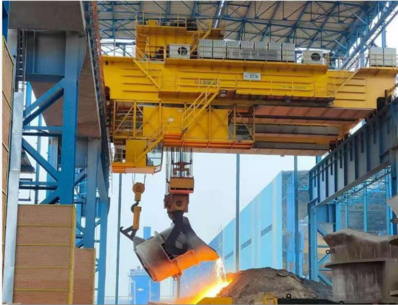
Anyang Steel & Iron Project
